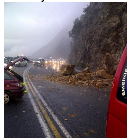
Photograph B – Rock fall on Sir Lowry's Pass
